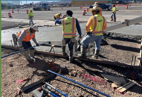
Sidewalk installation near Warm Springs Rd & Boulder Hwy
