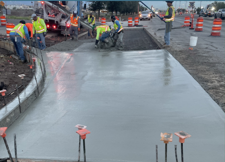
Driveway installation near Sunset Rd & Boulder Hwy
