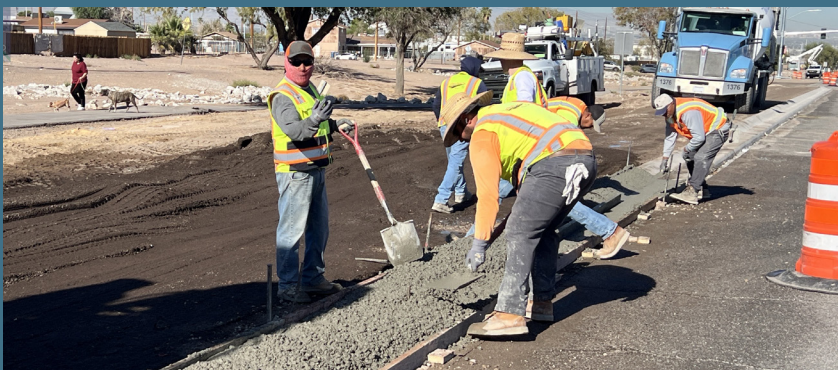
Installation of new curb
