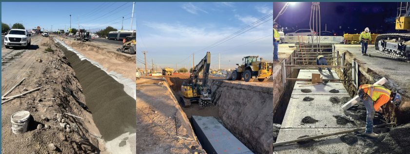
Storm drain improvements installed as part of the project
