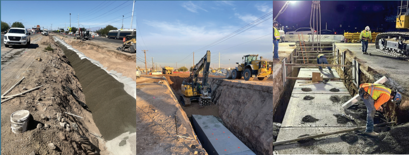
Storm drain improvements installed as part of the project
