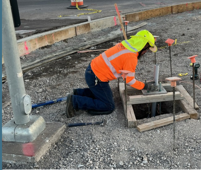
Crosswalk button foundation installation near Water St
