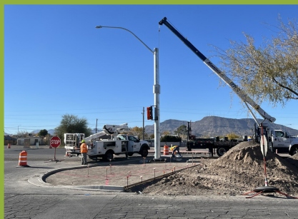
Crews placing a streetlight at the new access to Pioneer Rd
