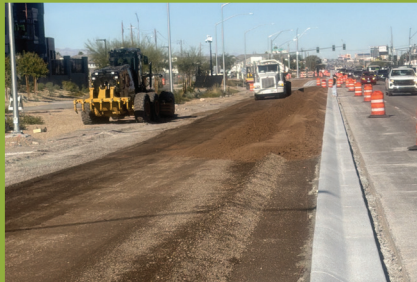
Grading of future cycle track near Gibson Rd
