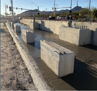
Concrete work for future bus stop at Magic Way
