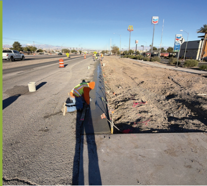
Curb installation near Lake Mead Pkwy
