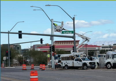
Street light installation at Galleria Dr
