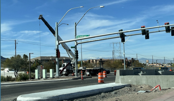
Equestrian Dr before: The new signal sits behind the old signal until it's operational
