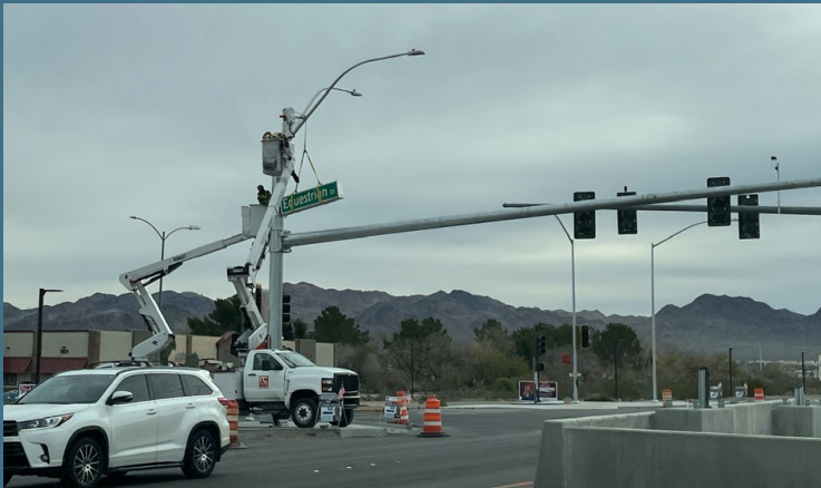
Equestrian Dr after: The old signal is dismantled and signage is replaced
