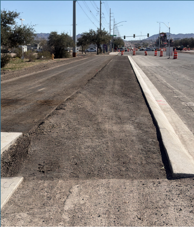
Future cycle track prepared for paving near Sunset Rd
